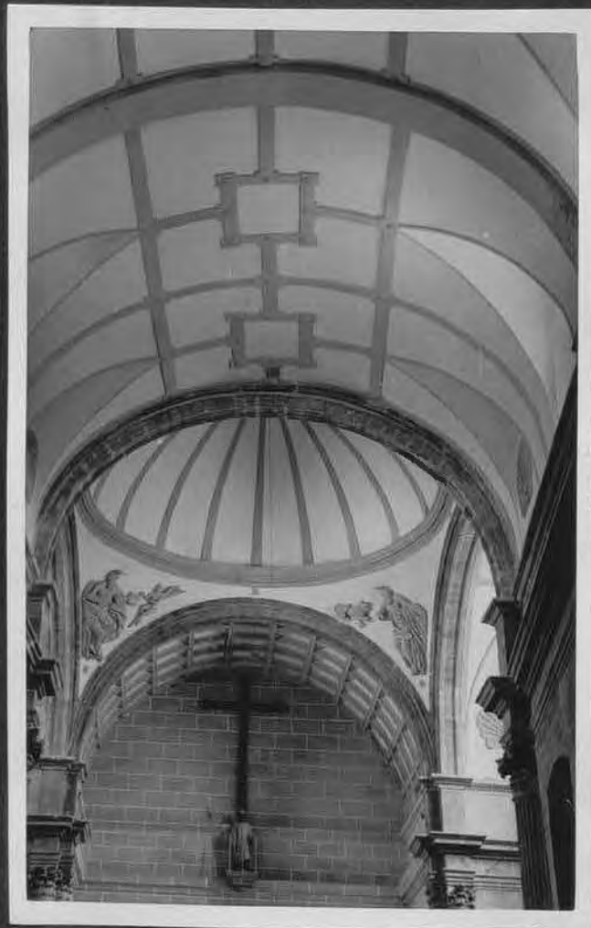
62 Ubeda - Hospital Santiago - Capilla
